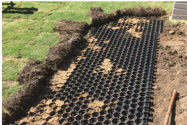
4. Spread sandy loam soil over the grid, with each hole in the grid filled with the soil.
