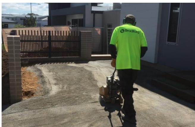
4. Spread sandy loam soil over the grid, with each hole in the grid filled with the soil. For this project a bobcat moved the bulk of the soil and then rakes were used by hand to spread the soil into each grid hole.
