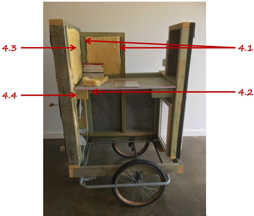
*Right side of the trailer: shows how insulation is typically installed.*
