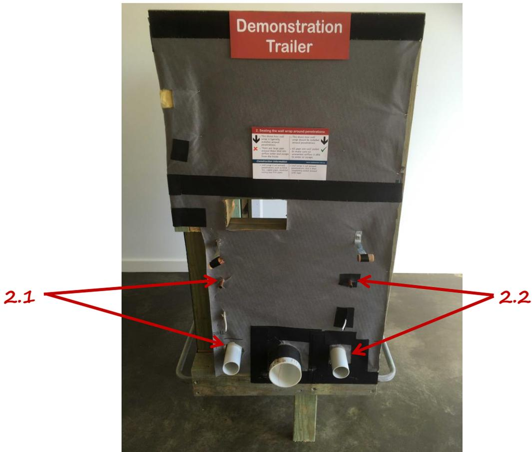
Left side of the trailer: shows how wall wrap is generally installed around penetrations.
