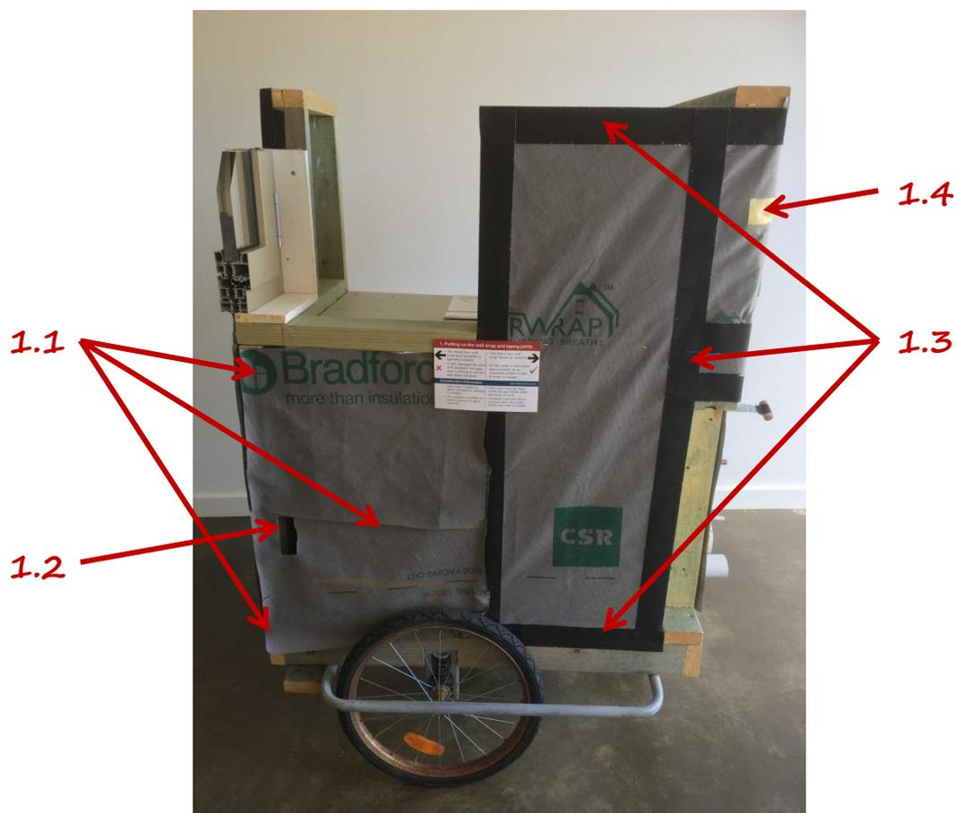
Left side of the trailer: shows how wall wrap is generally installed.
